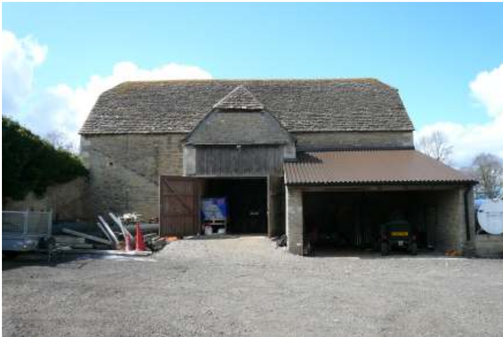
Eastern Elevation of South Barn (© Brian Clarke)
