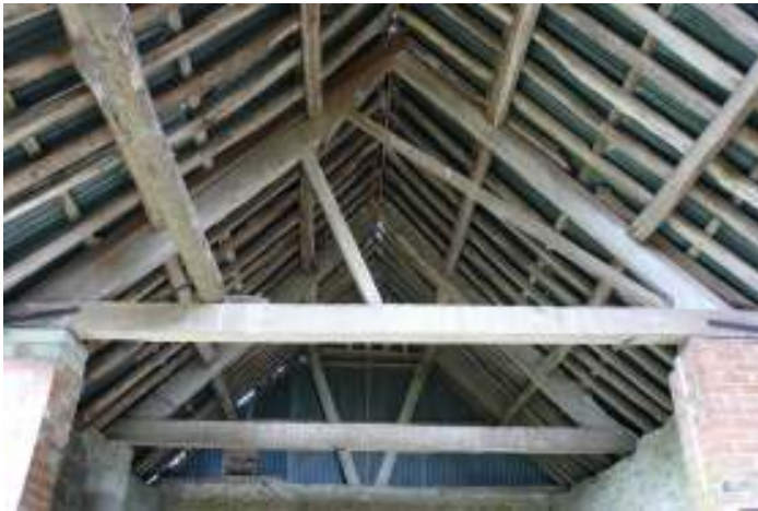
Figure 6. Barn Ground barn, Roof trusses, north end. (© Brian Clarke)
